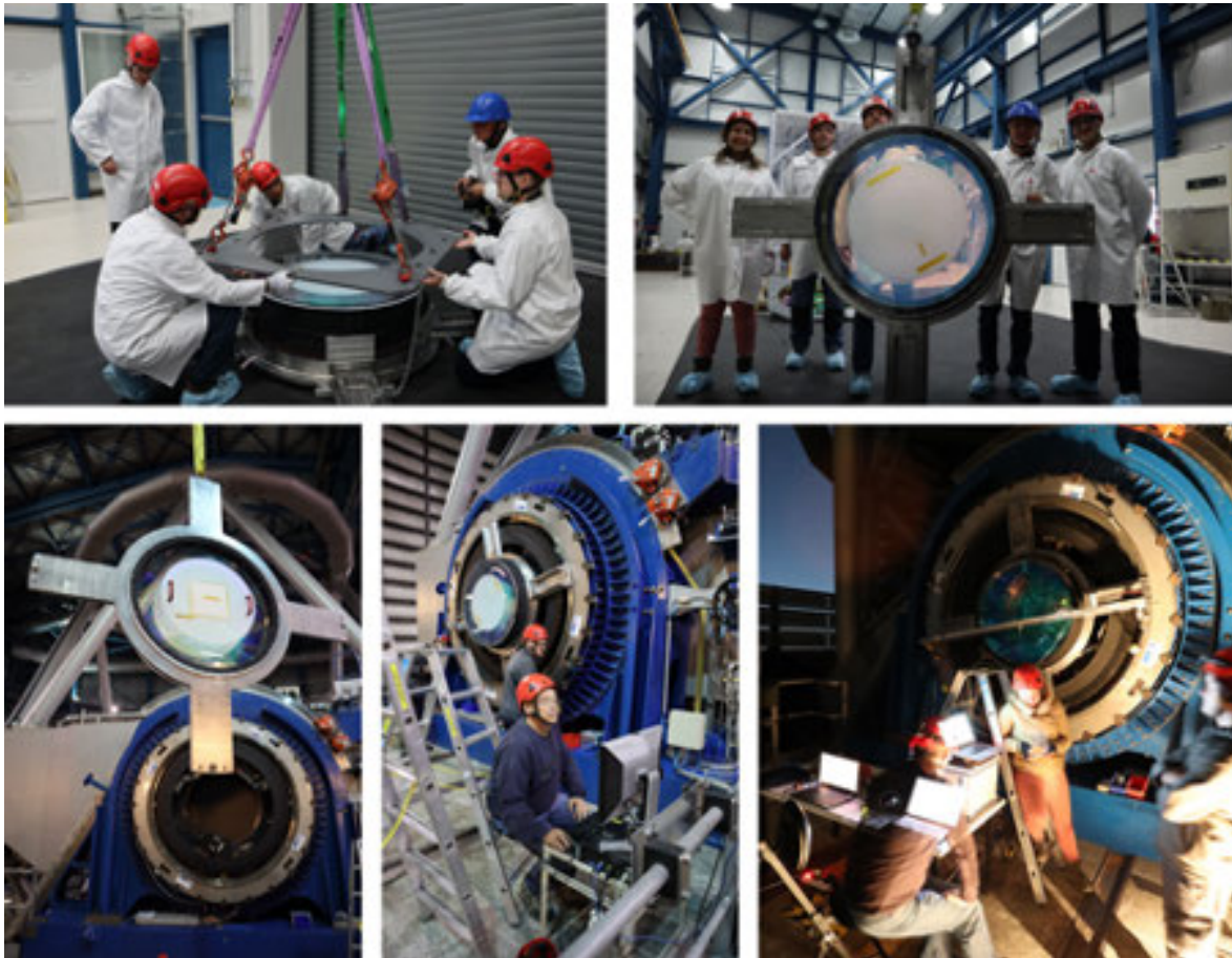
Figure: The MOONS (ESO) Field Corrector being installed in the ESO Paranal observatory.
