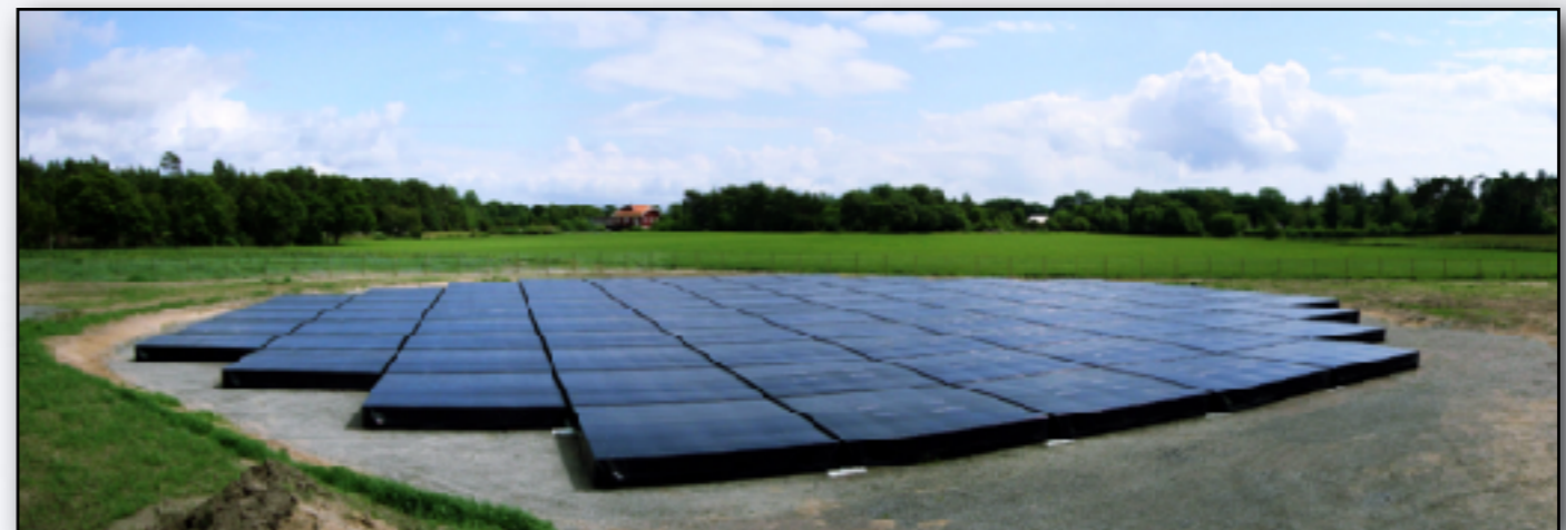
High-Band Antenna Station
