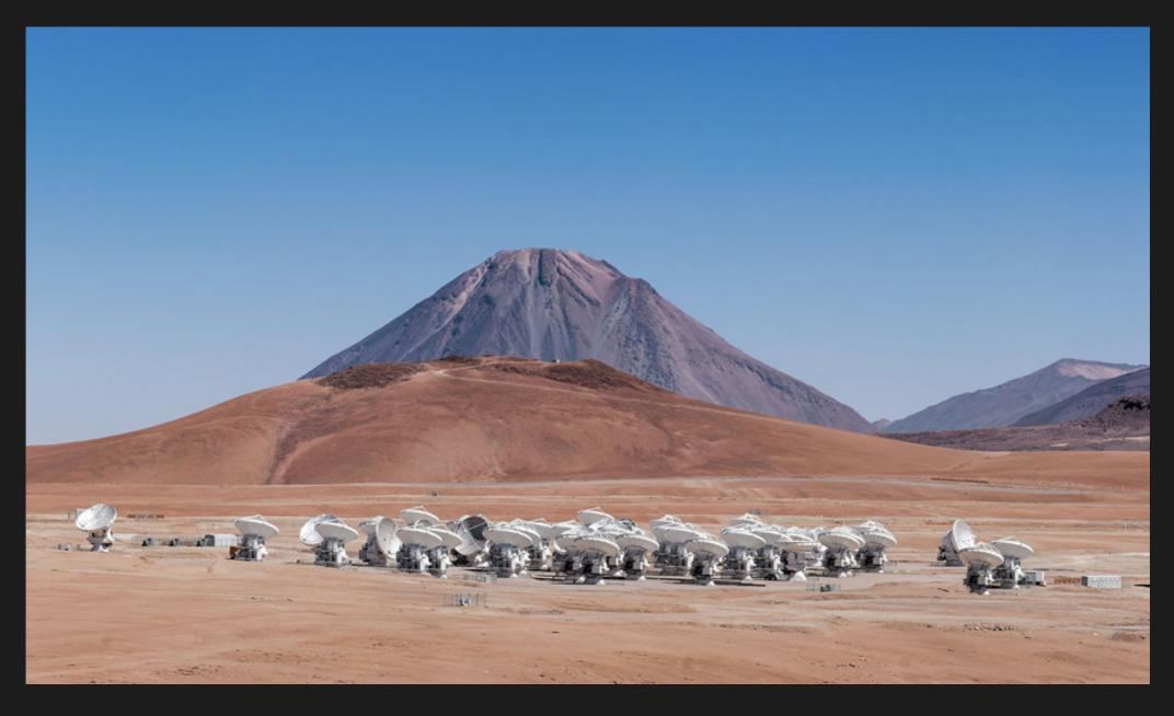
ALMA is a submm telescope designed to observe at 0.32-9.5mm (31-950 GHz)
